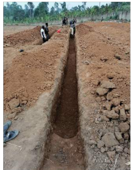
From Construction of Family Center Ghana
