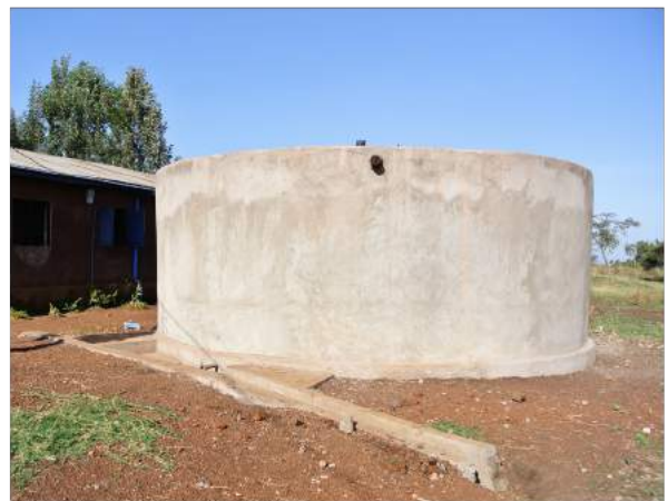
Primary school having a water tank built. Karagwe Tanzania, Mavuno
