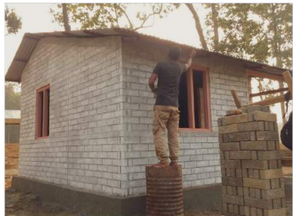
Process of making & using Earth Brick at BUN, Nepal
