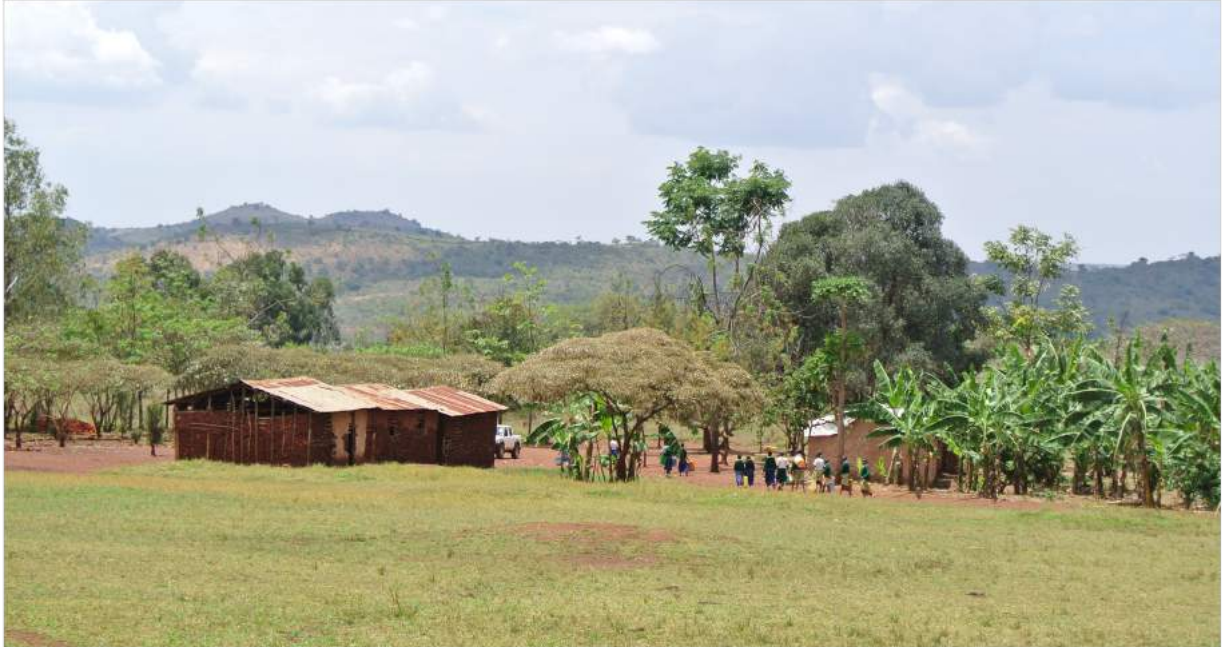
Primary school having a water tank built. Karagwe Tanzania, Mavuno
