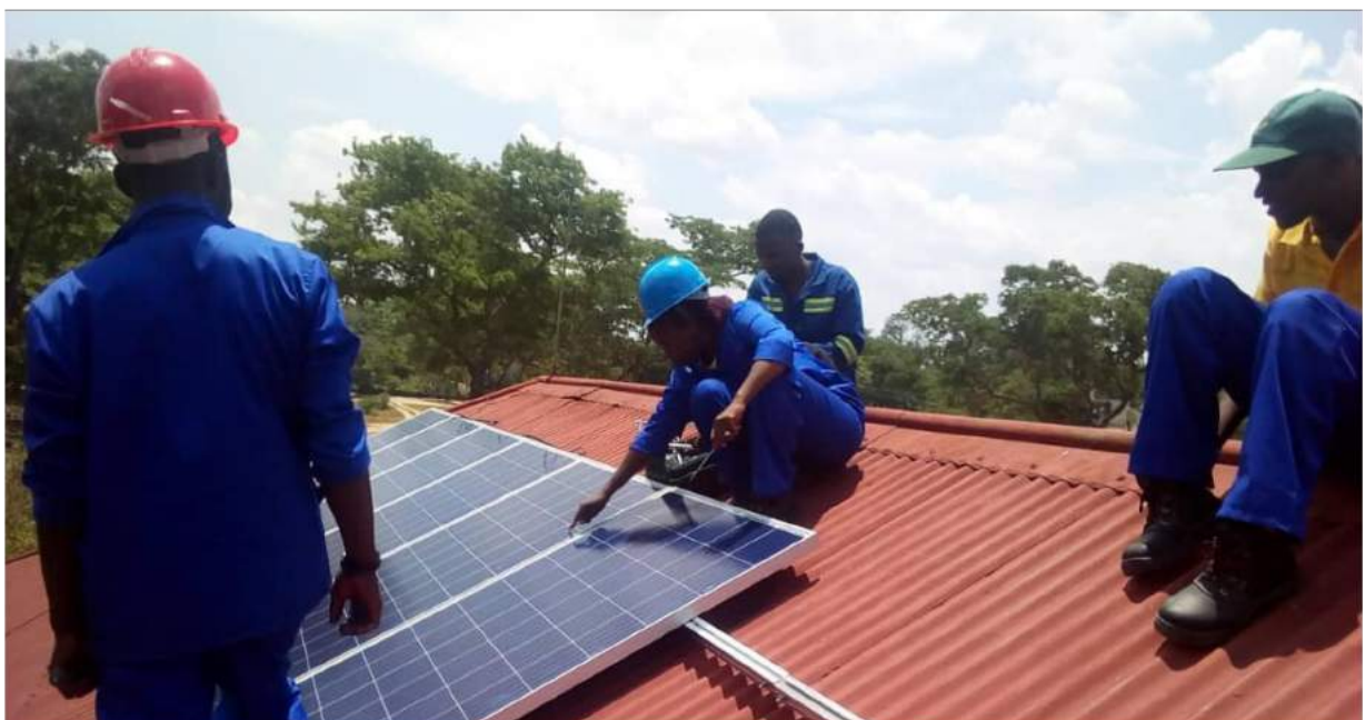
Installation of solar panels at Rusape Hospital in Zimbabwe
